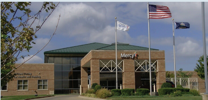
The former Mercy Fort Scott Hospital
